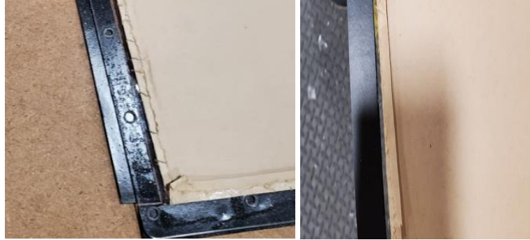
Figure 6: Taping edges of Door Window (Back and Front)
